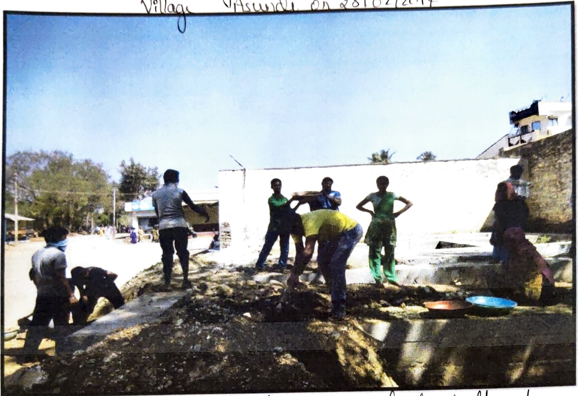
Nearly 6 Lorry of mud is dumped at plinth site
